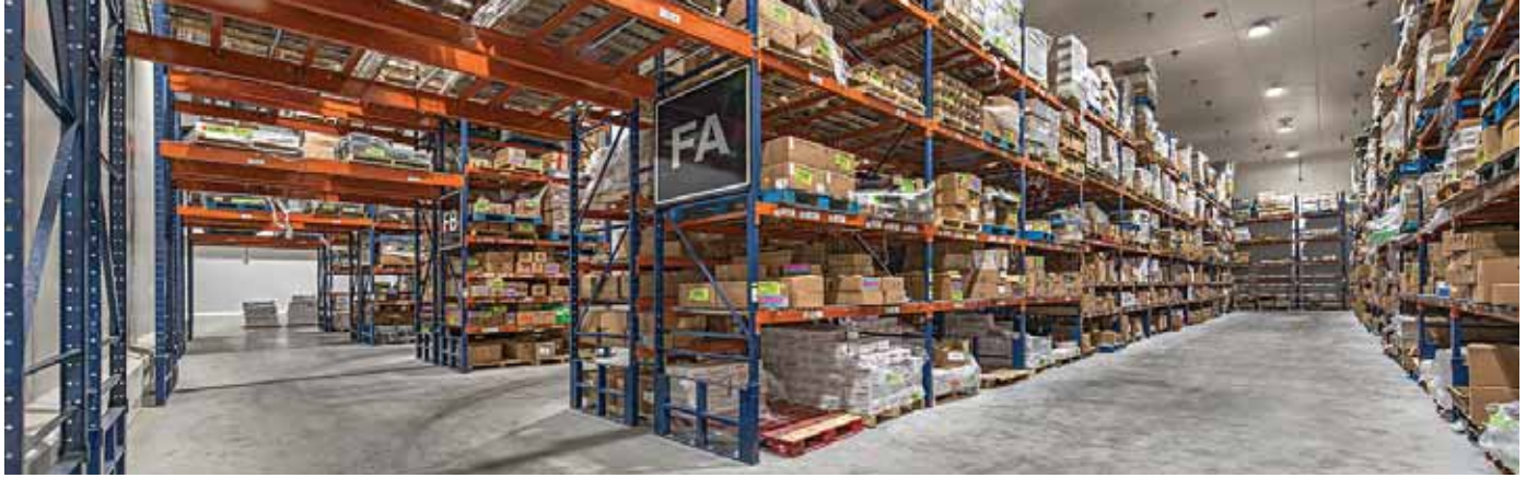
The original dry warehouse was converted to refrigerated storage and processing spaces with a system of insulated metal panel walls, liner panels, baffles and ceilings. (Photo courtesy of A M King.)
