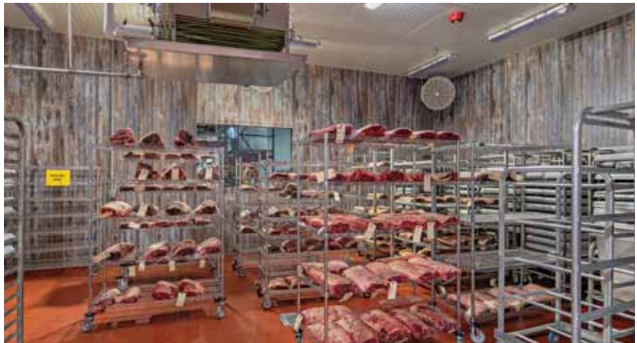
A distinctive 34-degree, 4,200-square-foot dry beef aging room is fitted with high-tech temperature and humidity controls and large viewing windows for customers. (Photo courtesy of A M King.)
