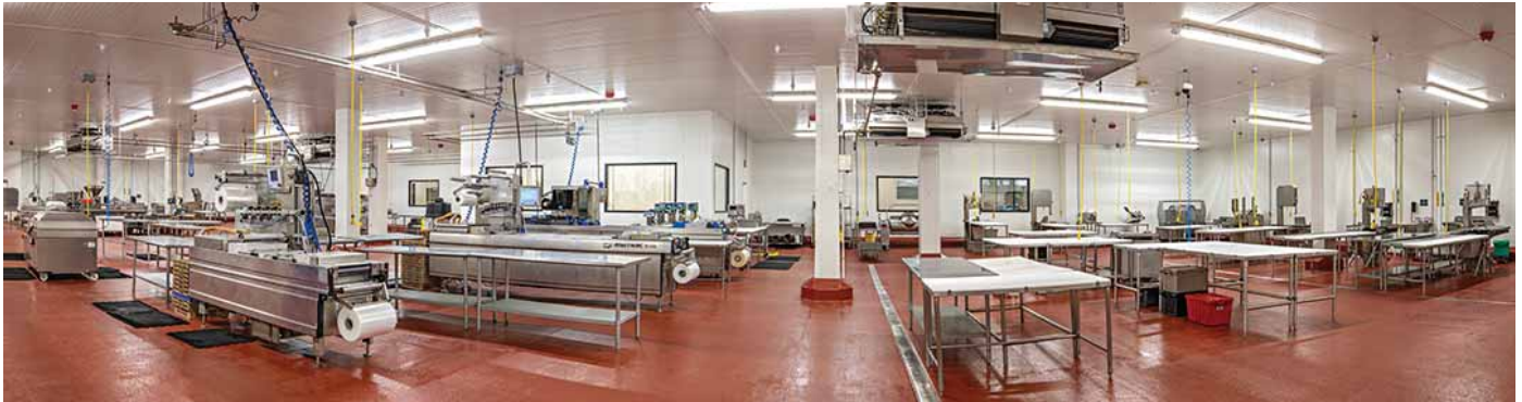
A high-strength industrial floor coating over all concrete slabs in the food processing area prevents food particles from absorbing into the concrete slab and minimizes the risk of bacterial growth. (Photo courtesy of A M King.)
