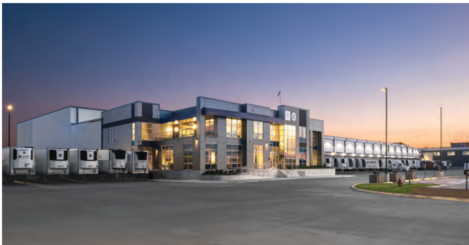
Primus installed solar-reflective materials to the U.S. Cold Storage facility in Covington, Tennessee, to ensure the building’s roof and paved areas do not create an irregular “heat island” in a rural setting. Light pollution was mitigated with outdoor fixtures that cast light downward and not beyond 15 feet of the property. (Photo courtesy of Primus Builders.)
