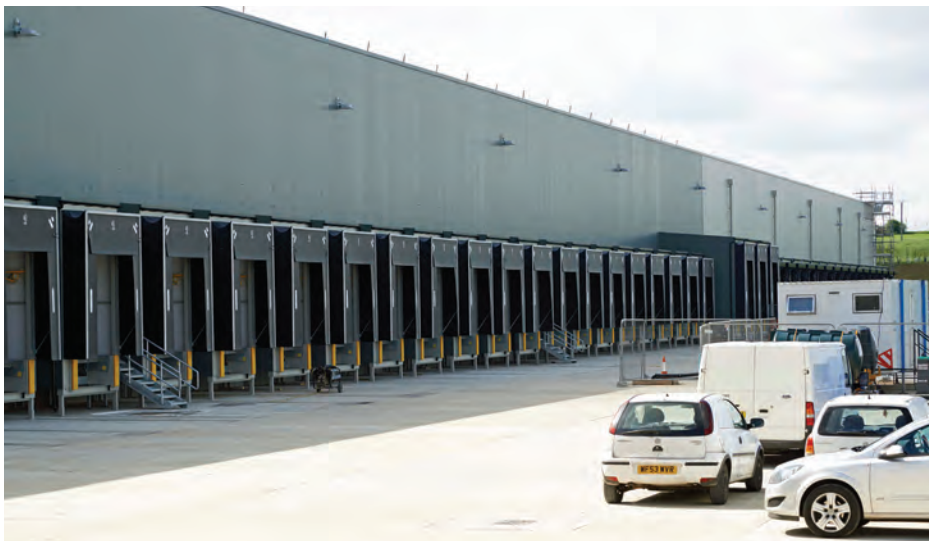
Aldi's new cold store and warehouse was built using ISD's single envelope construction to increase energy efficiency. (Photo courtesy of ISD Solutions)
