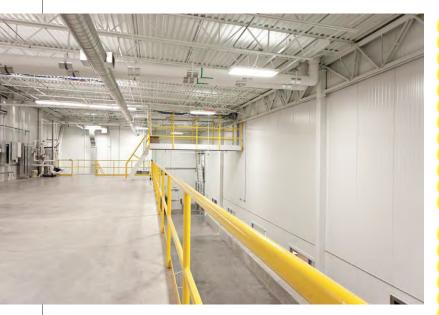
To minimize risk, forklift traffic routes should be kept separate from personnel traffic; interstitial spaces (access shown in rear) can be used for piping and conduits. Source: Curtis Waltz, Aerialscapes. each project subcontractor a copy of "Gray's Contractor Guidebook for Food Plant Construction" to help ensure food safety and sanitary practices are followed.
