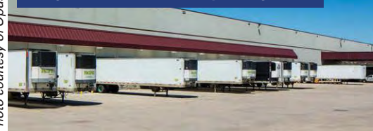
Opus completed its third expansion to Oneida Cold Storage's Henderson, Colo., cold storage facility, which is a state-of-the-art, high-cube refrigerated foods and grocery distribution center offering refrigerated, frozen and dry storage.
